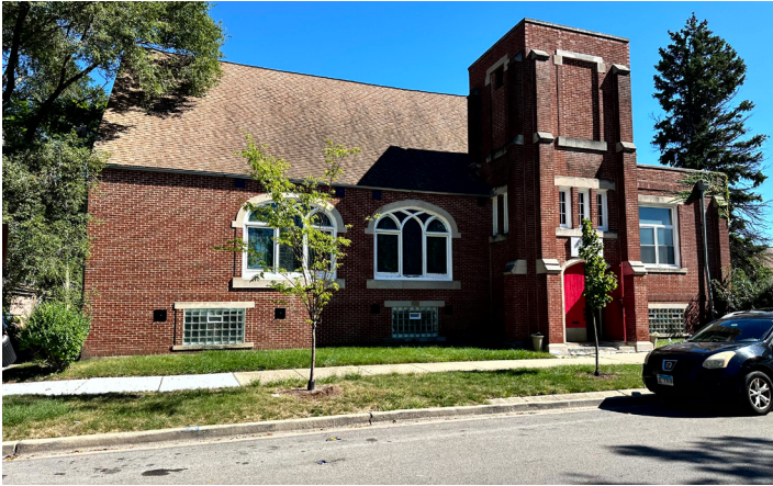
EXTERIOR FROM S SANGAMON STREET
